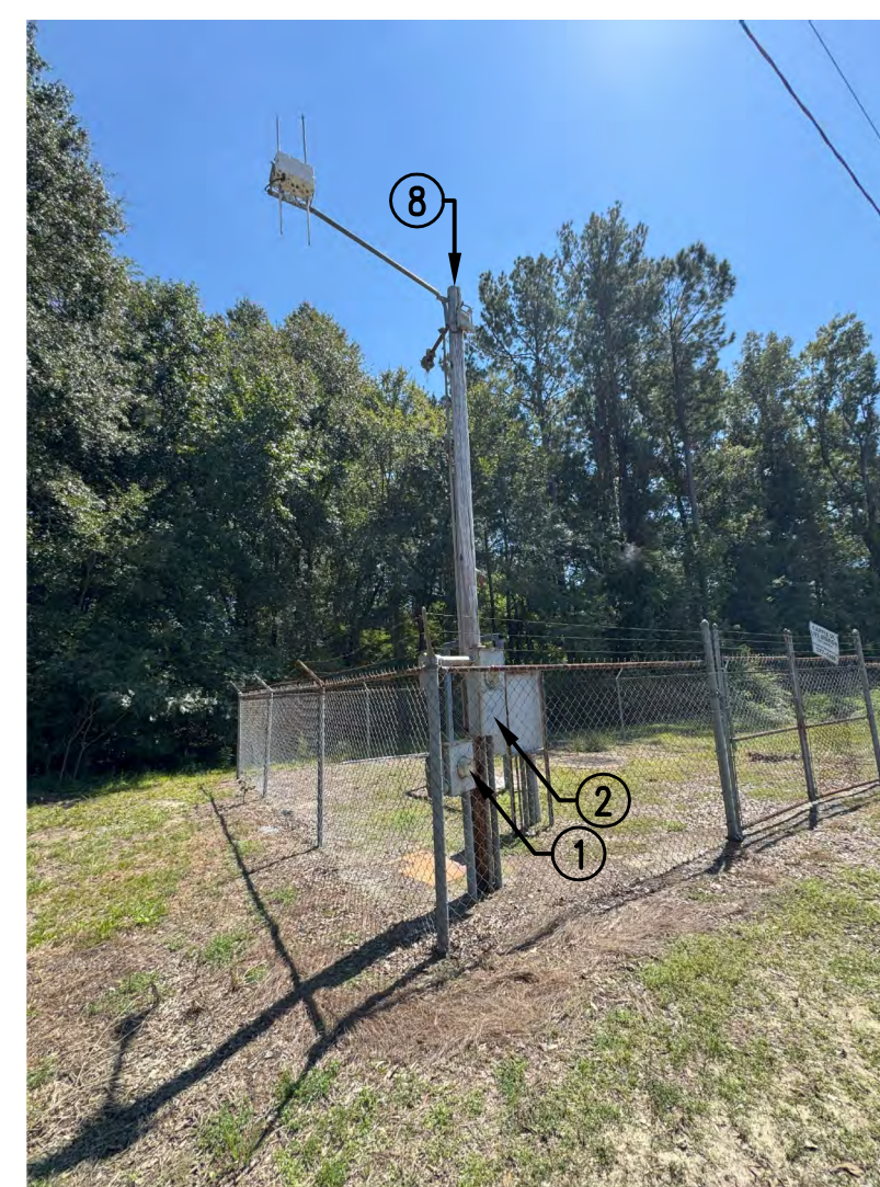
EXISTING CONDITION PHOTO 2 SCALE: NONE
