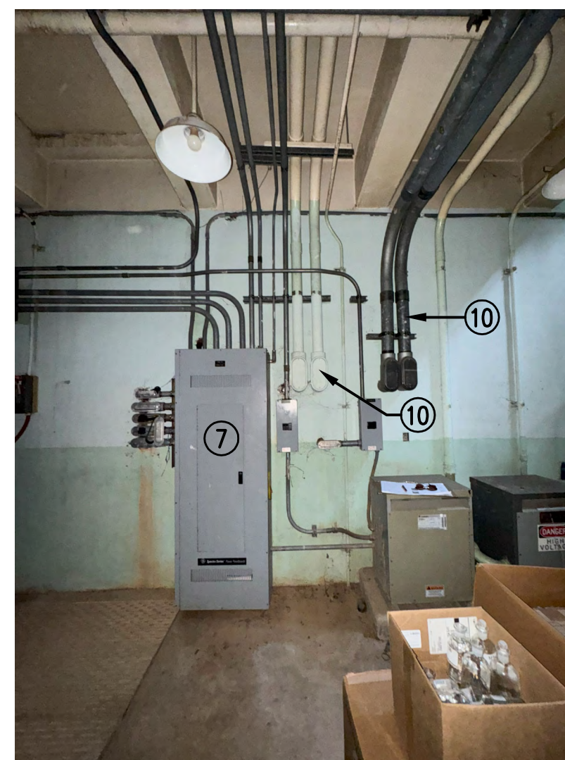
EXISTING CONDITION PHOTO 2
