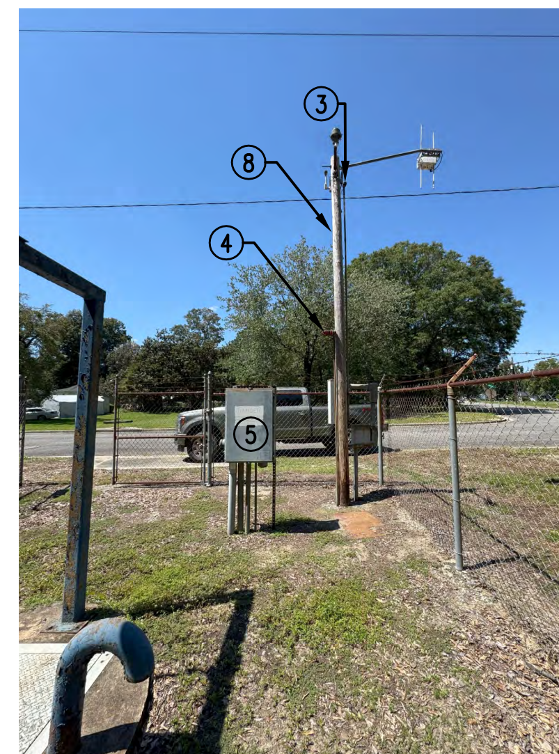
EXISTING CONDITION PHOTO 1 SCALE: NONE
