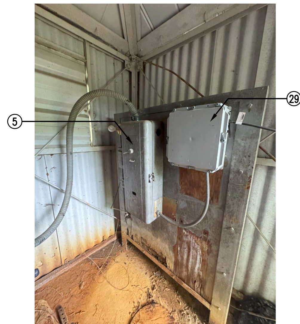
EXISTING CONDITION PHOTO 1 SCALE: NONE
