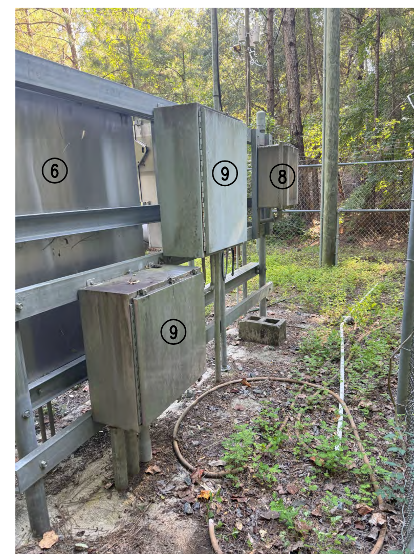
EXISTING CONDITION PHOTO 2 SCALE: NONE
