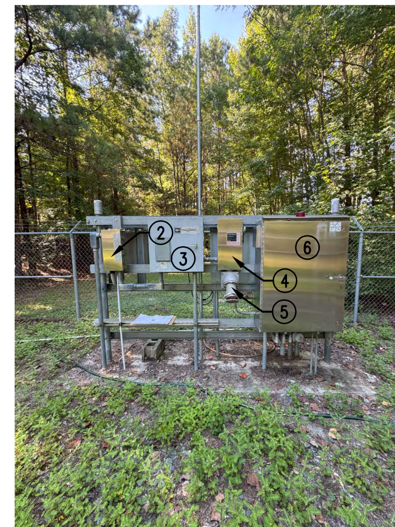
EXISTING CONDITION PHOTO 1 SCALE: NONE
