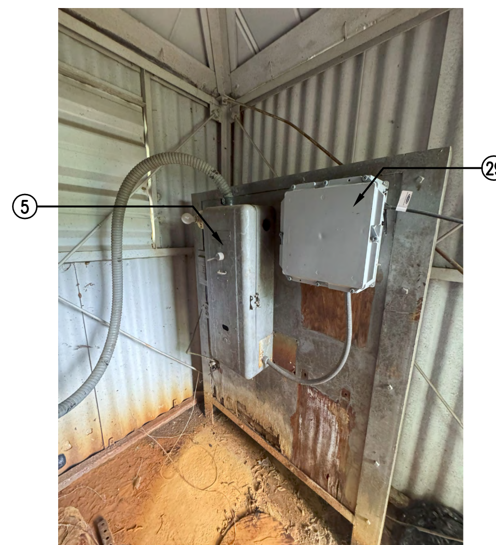
EXISTING CONDITION PHOTO 1 SCALE: NONE
