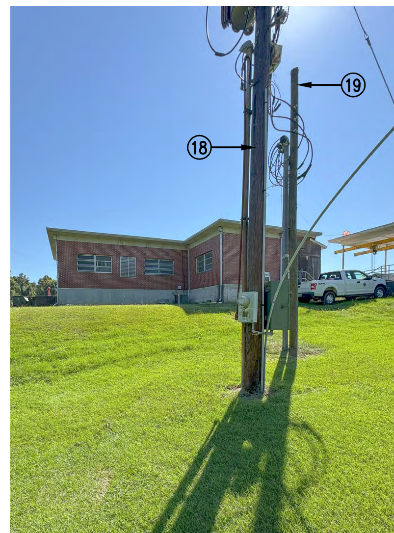
EXISTING CONDITION PHOTO 1
